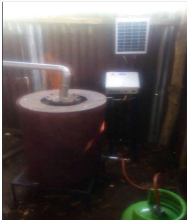
Figure 2 Gas-fired furnace with attached solar-powered temperature sensor
