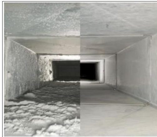
Figure 3 Internal View of Dirty-Clean Ventilation Channel [50].
